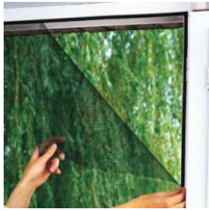
Mosquito screen to repair
